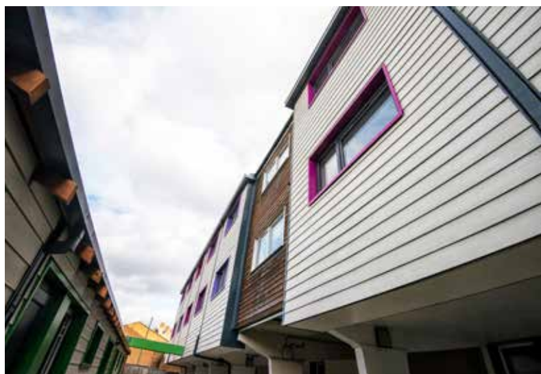
Nottingham City Homes: Energiesprong Retrofit, Melius Homes
